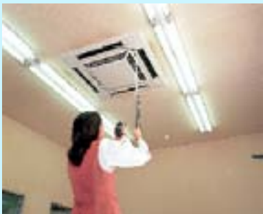
Check airflow rate of air conditioner
