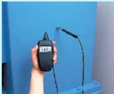
Measuring airflow rate inside duct
