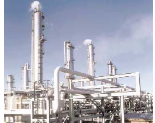
Figure 1: Catalytic reformer in a refinery
