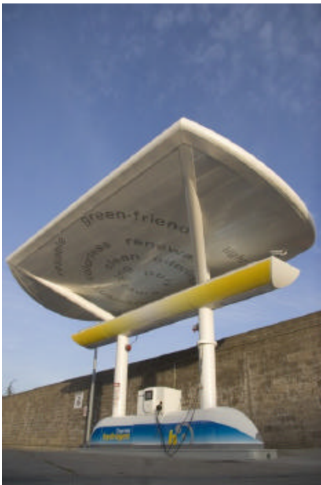
Fuel Cell Station
